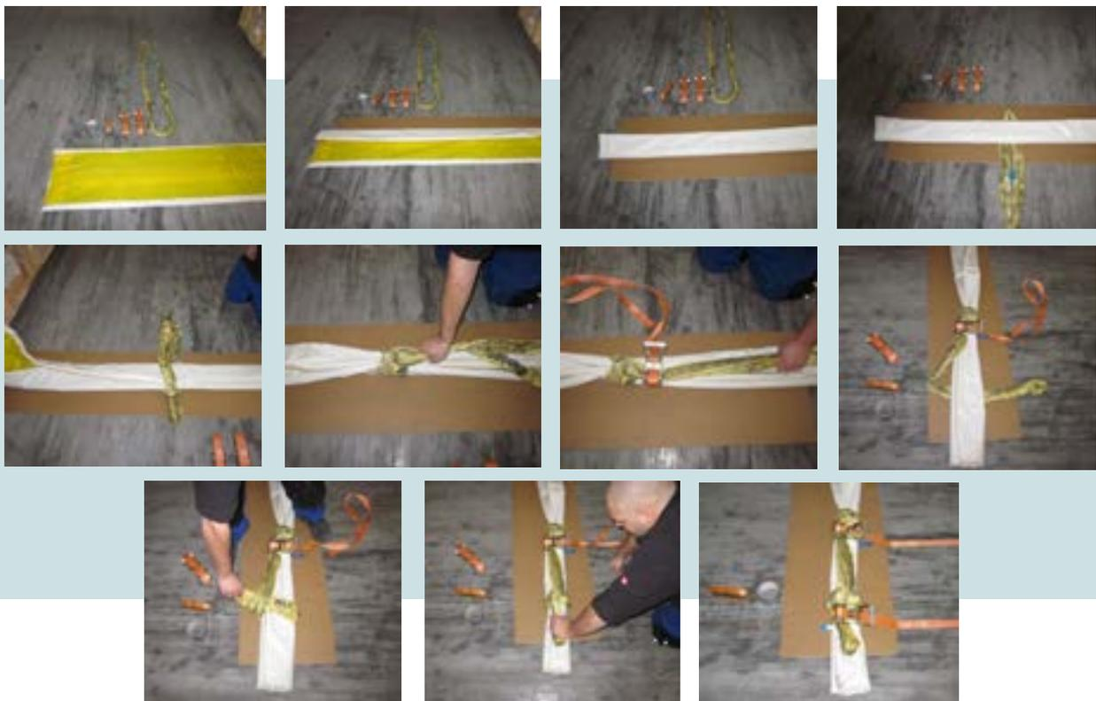
The IMPREG<sup>Liner</sup> must be folded to half its original width before being fed down into the manhole. The folded liner is then lowered to a worker in the manhole. This worker guides the liner into the pipe and monitors to make sure it is going in correctly. The end of the liner can be lowered in with a rope depending on the depth of the manhole.
