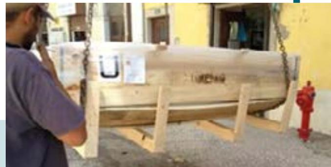
*Pulled-out nails due to the forklift forks being too short to support the entire width of the crate.*
