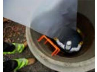
The sliding sheet must be fixed in the insertion manhole under an inflatable pipe plug placed in the opposite manhole or, alternatively, fixed to the bottom of the manhole by means of floor anchors. This sheet protects the IMPREG<sup>Liner</sup> as it is inserted into the damaged sewer section, allowing the liner to slide easily along the bottom of the host pipe.
