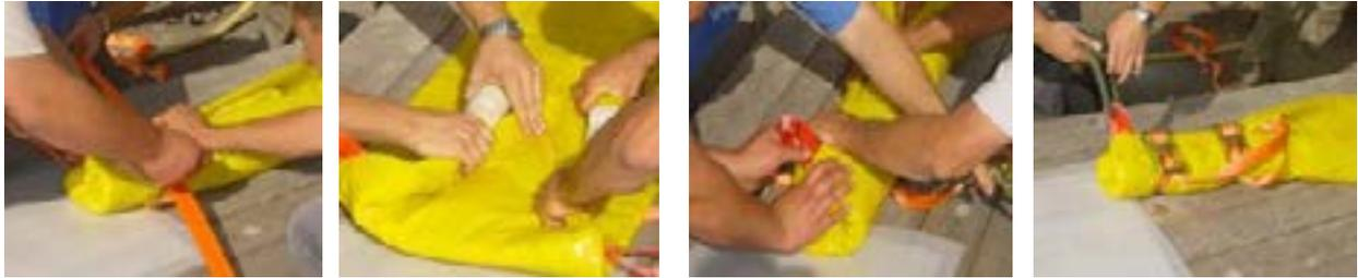
*Conventional method - binding the pulling head using 2-3 lashing straps*
