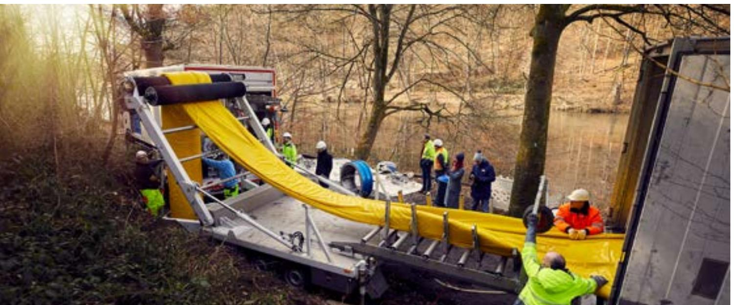
If the IMPREG<sup>Liner</sup> is to extend through multiple sewer sections, a worker should check that the liner is being pulled past the intermediate manholes correctly.
